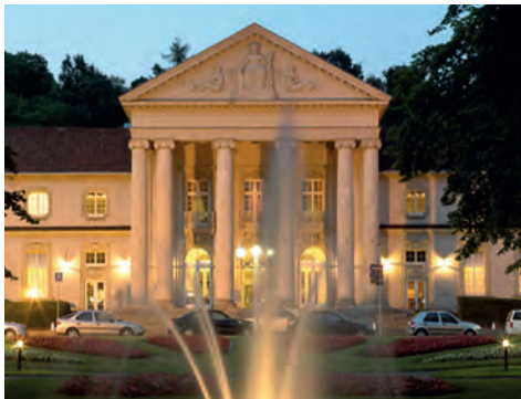
Neues Kurhaus/Casino Aachen | New Spa House/Aachen Casino
