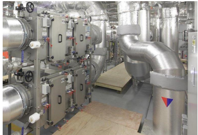
HEPA – filter systems on the filter floor of the laboratory
